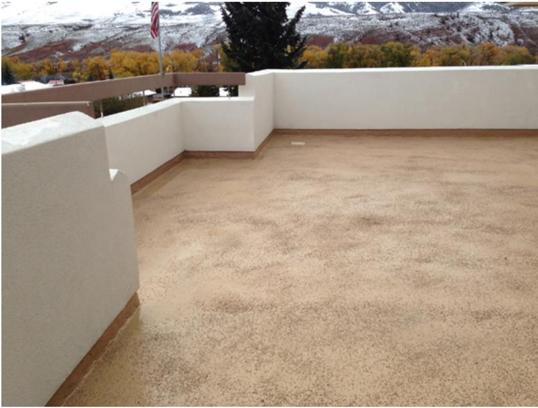
After the joints and cracks were completed and cured a ph test was performed to assure surface was ready for primer.
