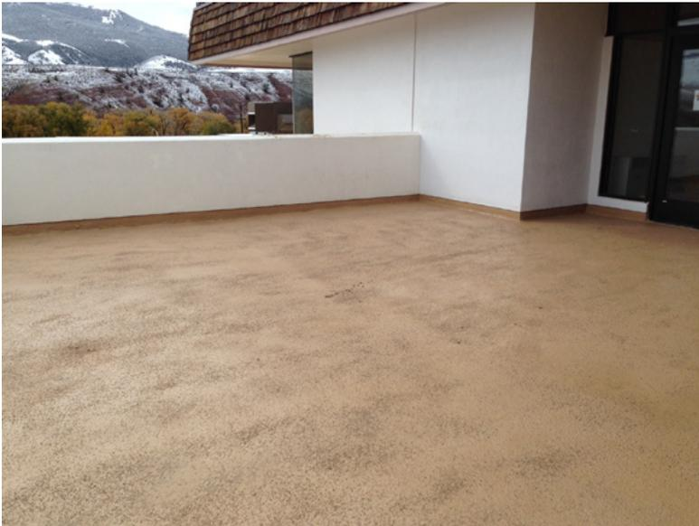
380 with crumb rubber, the coating was allowed to cure for a short time so they could walk on it and perform the final application, which was to top coat the VF 380 with WB 252 (tan) for color stability.
