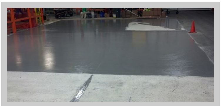
Initial Application, Warehouse Floor
