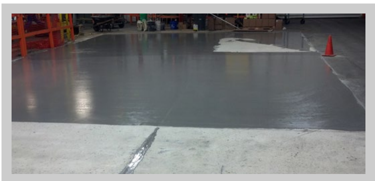
Initial Application, Warehouse Floor
