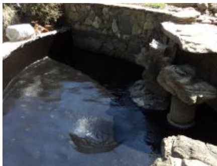
Koi Pond during and after installation of SL/75 using low-pressure spray equipment
