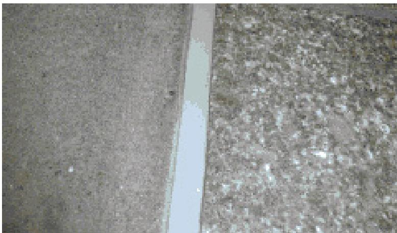
The installation contractor first attacked the deteriorated sidewalk by conducting typical concrete repairs, fixing radius-ed edges with new saw-cuts, and cleaning and prepping the concrete for optimum performance and adhesion of the joint fill material.
