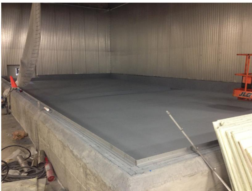
When the world's leading soup company needed a new durable, water resistant floor, it was a simple choice to select pure polyurea. When making soup for their famous "Ready to Eat" soup line, the final process involves the packaging into the cans. The soup is actually pre-cooked in the factory and immediately packaged. As a result, the soup cans get very hot and require a cooling cycle.
