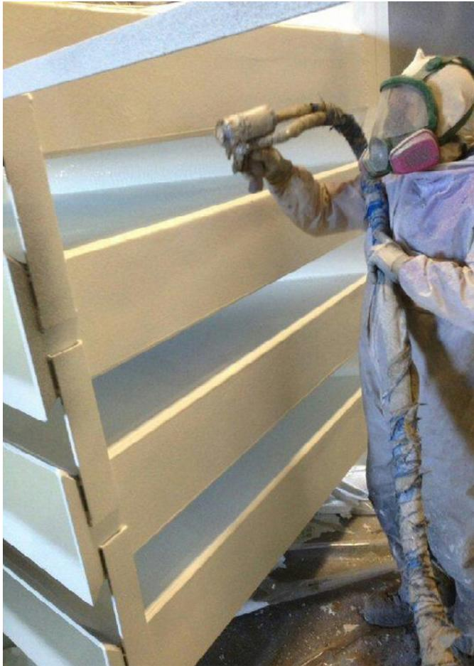
When a large Coal Mining Company in British Columbia, Canada needed to solve an abrasion issue in a coal hopper, they replaced the old epoxy system and turned to VersaFlex VF-330 Pure Polyurea and Spray All Poly, Ltd to solve their problems.
