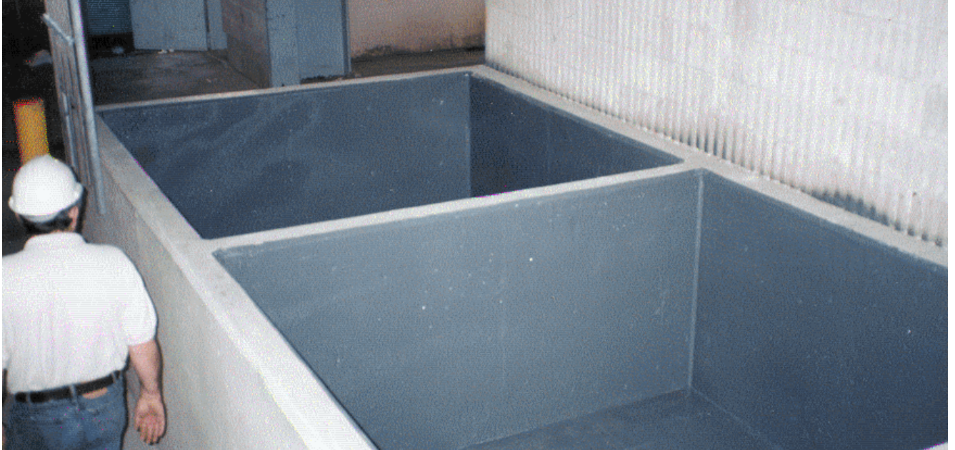
Preparation, Installation, Clean-up, and turn over was completed in only 2 days.
