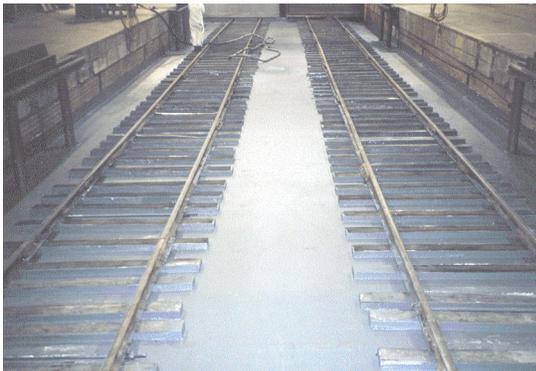
The floor was cleaned. Rail ties were grouted in place and doweled to prevent future movement. Ties were cleaned with grinding disks to develop mechanical bond. VersaFlex 45DC was sprayed at 60 mils over the cleaned floor and the rehabilitated ties up to the flat tie tops, allowing the ties to breathe during the change of seasons, since they could not be completely dried. This also allowed thermal expansion and contraction without restraining the stresses.
