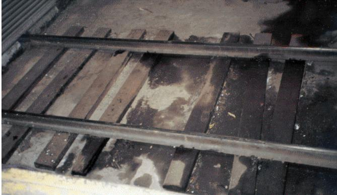
The massive Bowater pulp and paper facility at Thunder Bay, Ontario is utilizing polyurea to a greater and greater extent. This train shed has caused problems for years. Water carried into the shed on rail cars and snow melting off the cars had saturated the concrete floor, rotted rail ties, and had percolated down into the locker room below causing leak-related deterioration, staining, and a generally unappealing condition.
