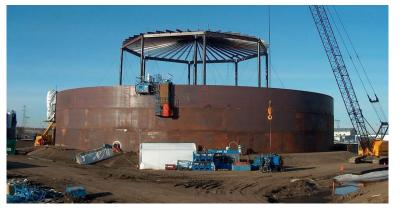
For Petro-Canada's GOT Project, two new chemical storage tanks were being constructed with a clay liner system for secondary containment. Petro-Canada and Stantec Consulting proposed a clay liner upgrade to a synthetic geo-membrane / polyurea based on the VF 380 pure polyurea elastomer system, as opposed to a sheet good liner system based upon a thermoplastic material. Being aware
