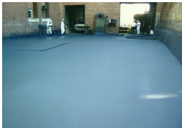
Finished installation of elastomeric waterproofing membrane
