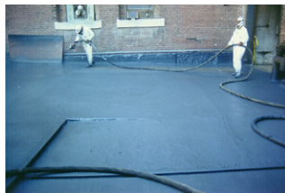
Application of primer and FSS 45DC spray polyurea (above)
