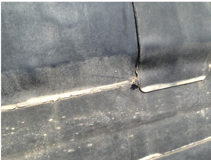
After completing the initial cleaning, a light hot powerwash with surface cleaner was applied to the roof while applying a bristle broom scrub to entire surface. This process helped to loosen and remove any oils, grease, etc that remained.
