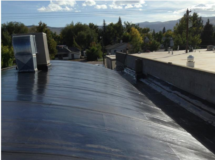
The customer, a commercial retailer in Wyoming, had a single-ply roof membrane with numerous cracks and seam separation, causing water to enter building.
