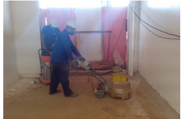
Surface Prep: Scarifying / Creating Profile
