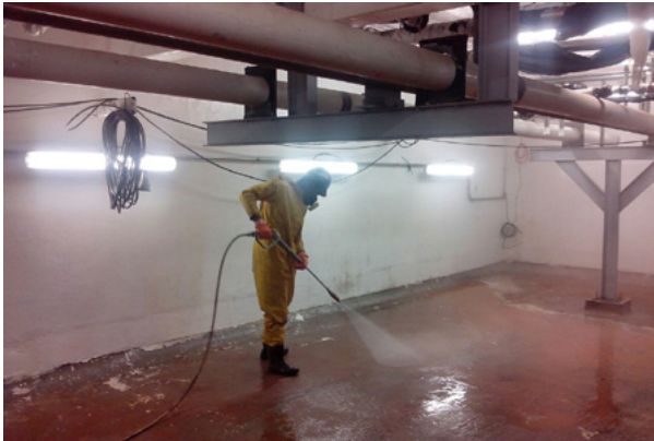
Surface Prep: Powerwashing
