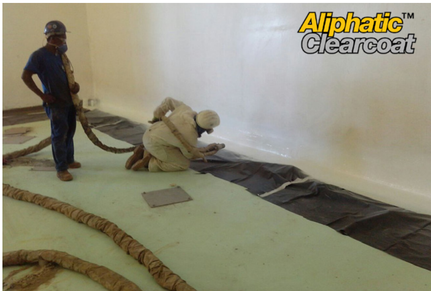
Coating Walls with Aliphatic Clearcoat™
