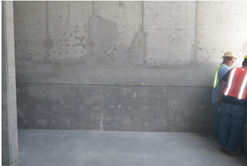
Termination Joint (saw cut)
