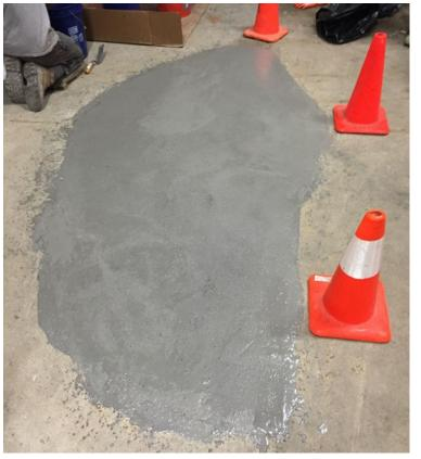
Due to the -20 degree temperature inside this freezer, it was not possible to make the repair with concrete. But Cassity had an alternative, VersaFlex's Quick Mender® X.O. concrete repair polymer, which was perfect due to its ability to fully cure in -20 degree temperatures and specially designed for confined space concrete repairs such as this. In addition, the Quick Mender® X.O. provided the rapid return to service that the facility owner desired.
