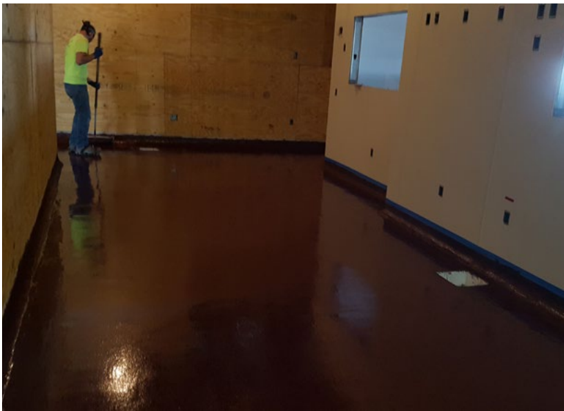
Epoxy coating install, kitchen area
