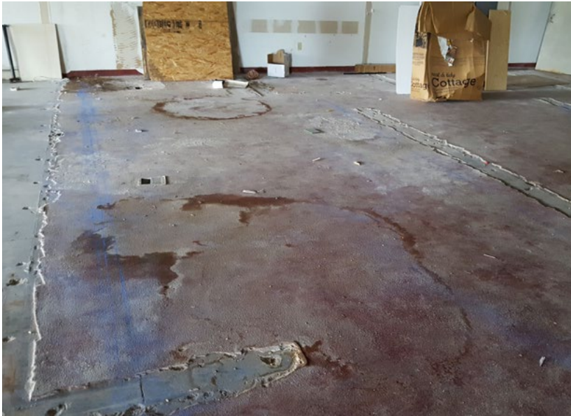
Initial view of the space with walls/fixtures removed
