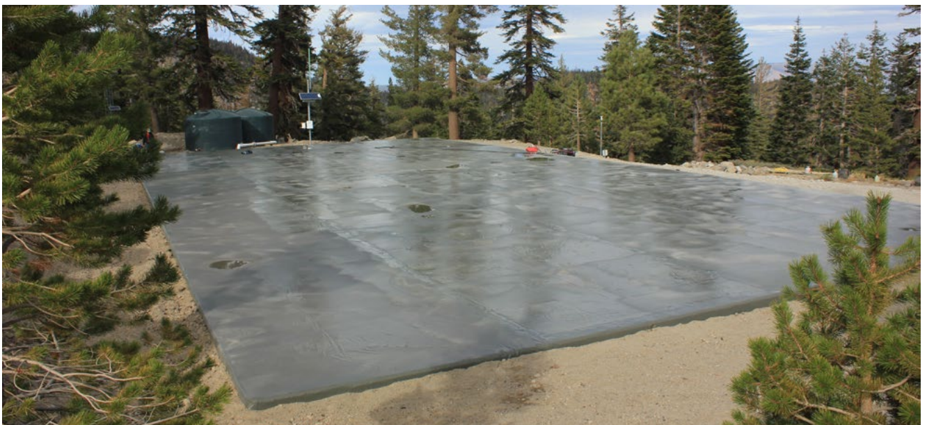
Finished Exterior Tank Top
