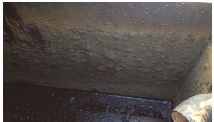
Existing Coal Tar Epoxy Coating
