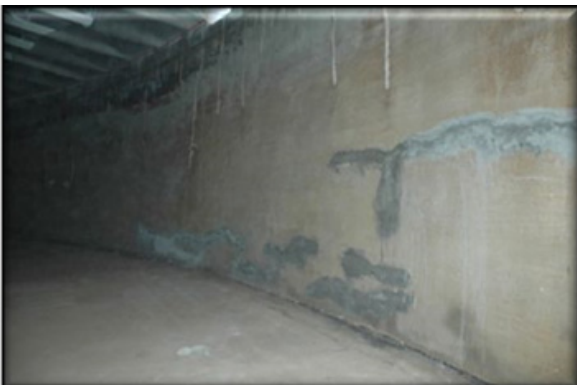
Cracks Repaired
