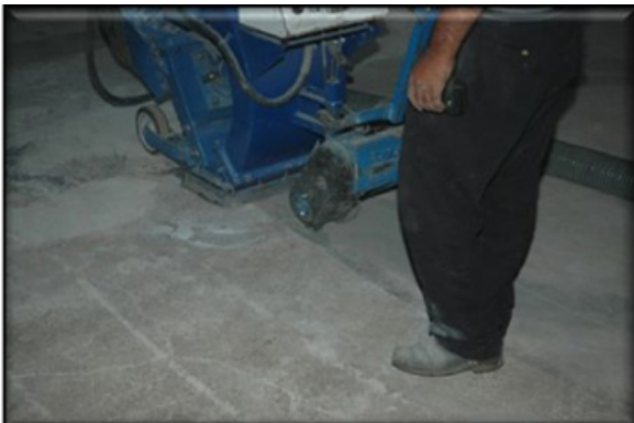
Shot Blasting Surface Preparation
