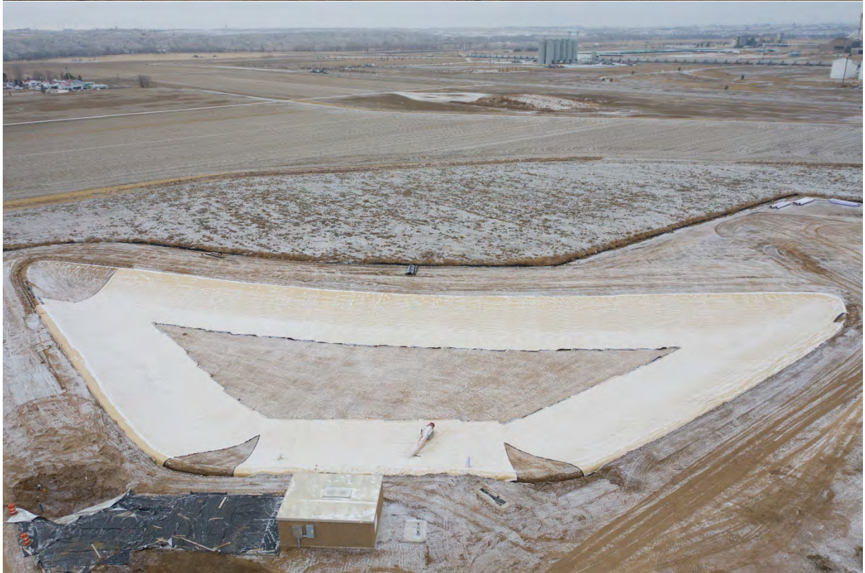
Installation progression Day 4 of 6 (top) – Snowy weather delay (bottom)
