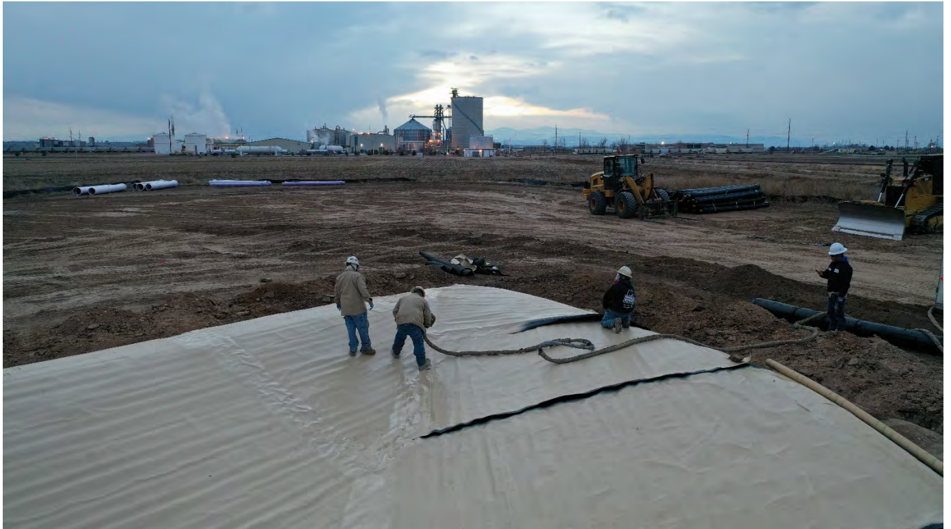
Panel Positioning (top) – Adhering the panel seams (bottom)
