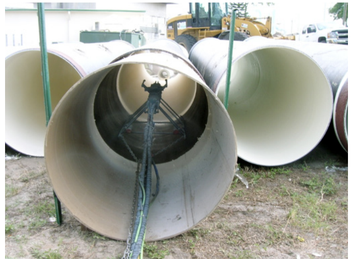
Figure 7: Lining Joint Sections of Pipe
