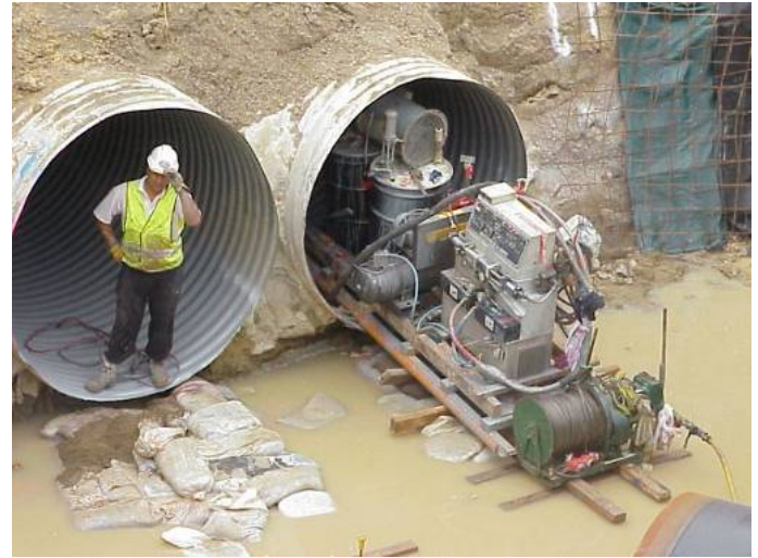
Figure 6: Lining Galvanized Corrugated Pipe with Polyurea Spray
