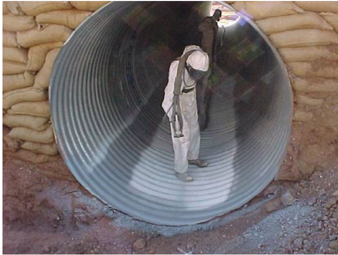
Figure 6: Lining Galvanized Corrugated Pipe with Polyurea Spray
