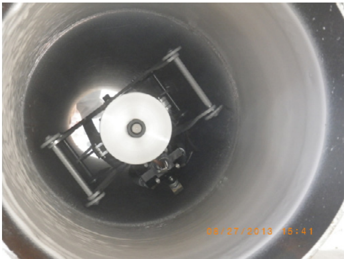
Figure 10: Commercial PUA Pipelining Spray Head, Spinning Cup & Static Mix
